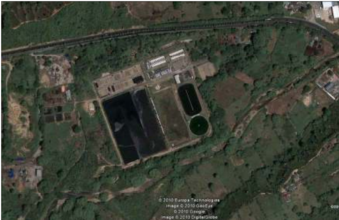
Figure 2.5: Satellite view of Río Frío WWTP in 2010. Source: [Google earth].
