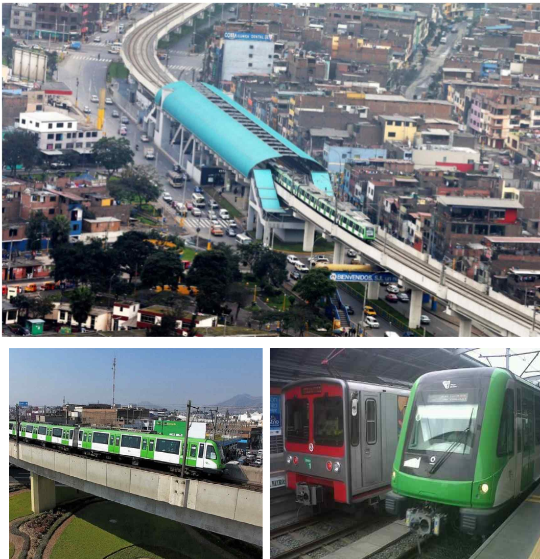
Fig. 4.7 Metro Line 1 views
