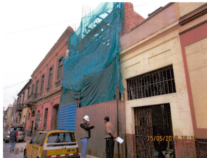
Picture 20. Inspection of 15 May 2019. Photograph by the Ministry of Culture.
