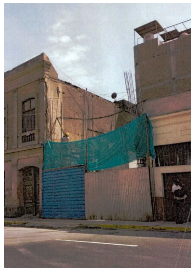
Picture 19. Inspection of 24 April 2019. Photograph by the Ministry of Culture.
