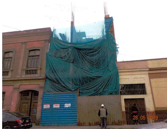
Picture 21. Inspection of 28 May 2019. Photograph by the Ministry of Culture.
