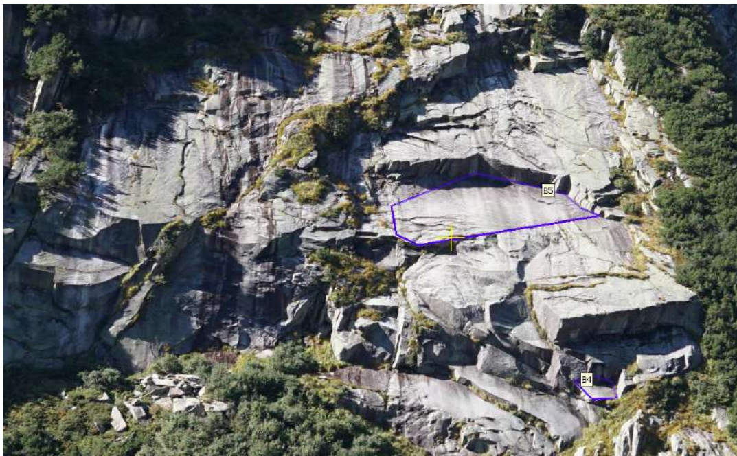
FIGURE 5.14: Handegg: Same area shown in Fig.5.13. Showing two failed blocks that were identified. They are limited with a violet polygon. There is a central one and the other is in the bottom left part of the picture.
