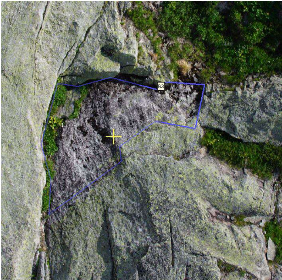
FIGURE 4.14: Failed block (B3) from Lake East. It is possible to identify the area where the block was due to a brighter coloration of the Granite.
