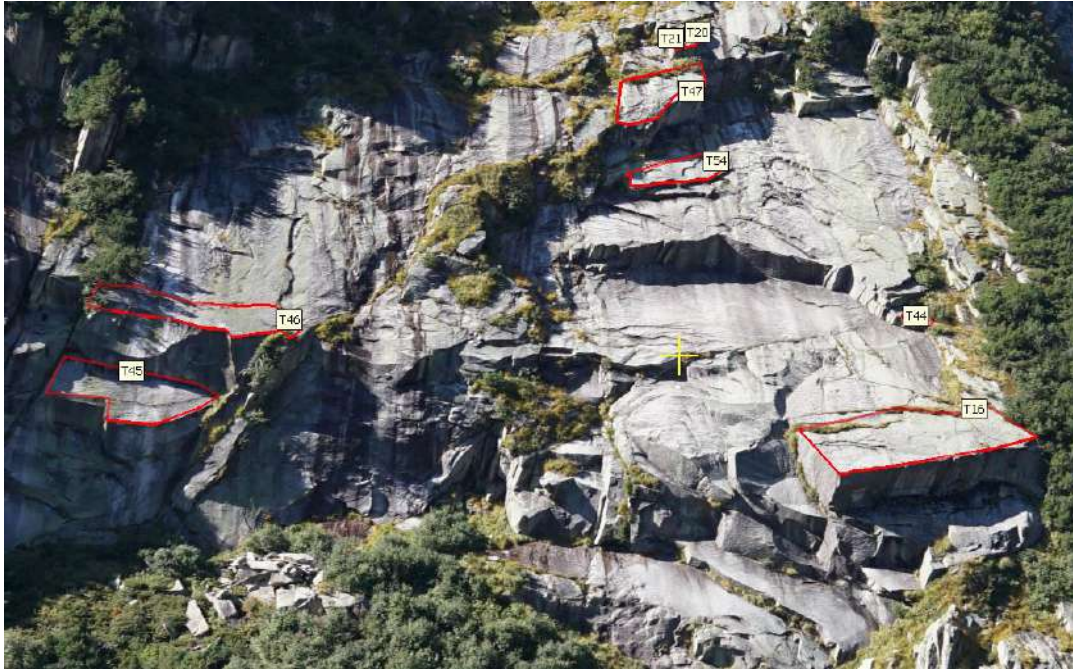
FIGURE 5.13: Handegg: Close-up to see the existing blocks.
