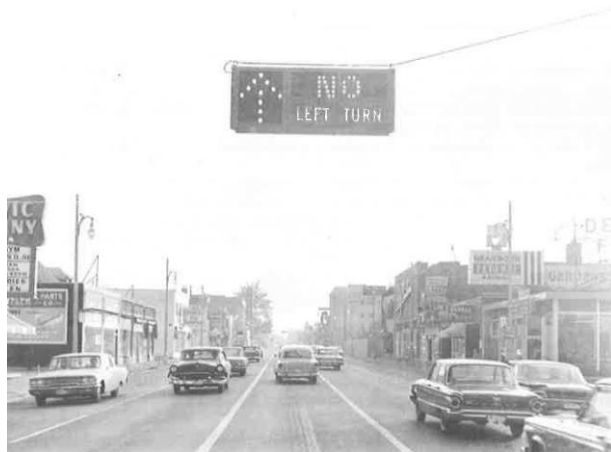
Fig. 4 Reversible center-lane signal; green arrow for center-lane usage [32]
