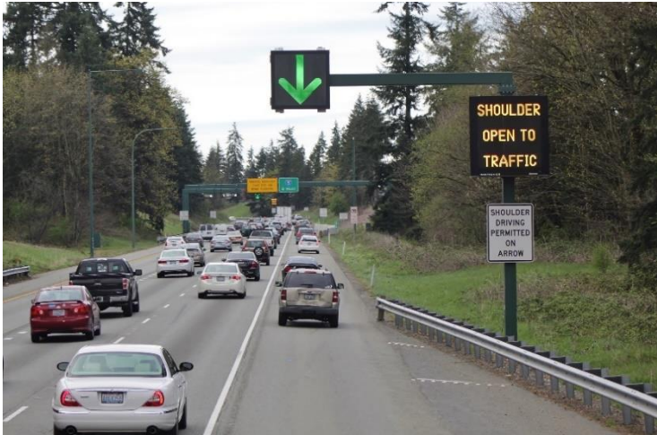
Fig. 2 Interstate 405 northbound shoulder bypass near Bothell, WA [13]
