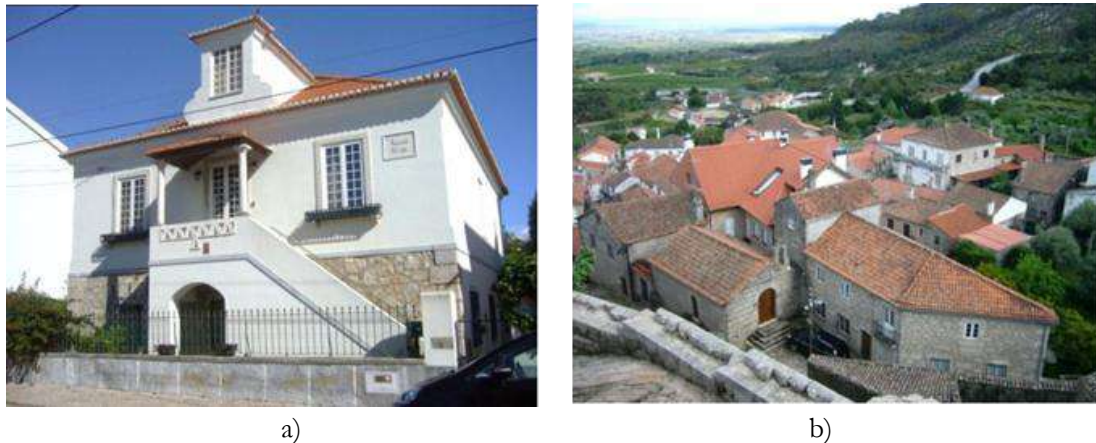
Figure 2.4 Examples of unreinforced masonry buildings: a) limestone and b) granite [57]
