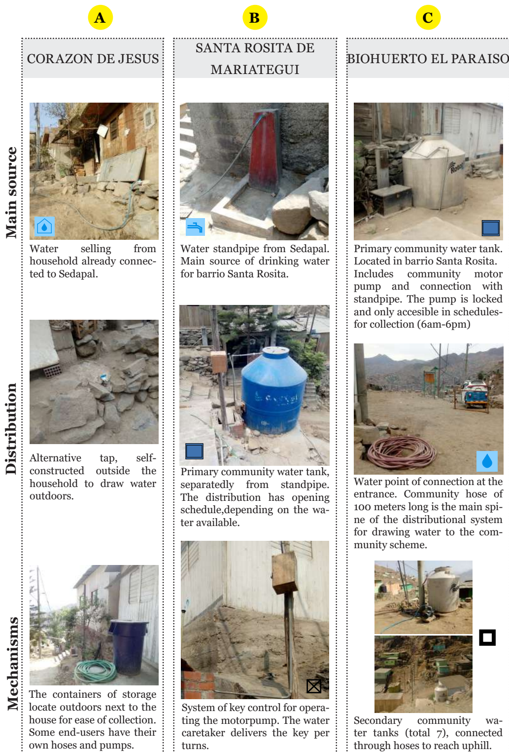
Figure 5.3 - Technological arrangements in community-led system for access to water (poly-tanks, booster pumps, public standpoint and hoses). Source: Author, 2020. Photography taken in March, 2020
