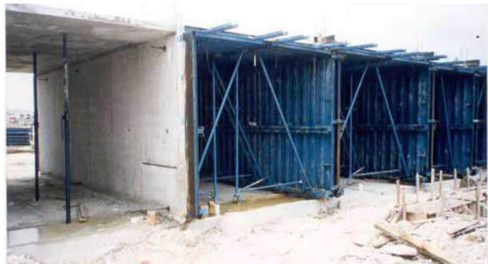
Figure 3.20. Monolithic structure with tunnel formwork
