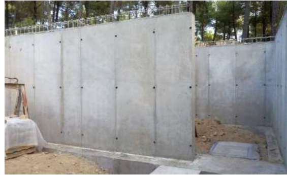
Figure 3.8. Wall poured until slab bottom
