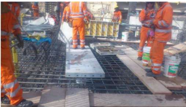
Figure 2.9. Formwork element used as a work platform
