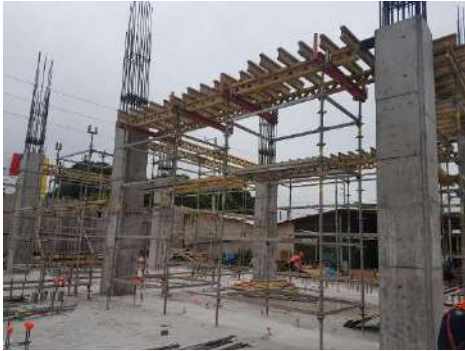
Figure 3.7. Column poured until beam bottom
