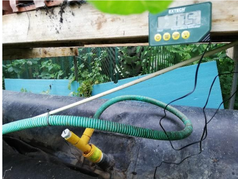
Figure 8. Extech TM20 Thermometer measuring the temperature inside the digester interior installed
