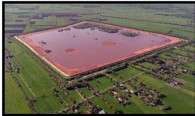
Figure 1.5 Tailings Dam - Ring Type ( http://www.wikiwand.com )
