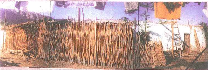
temporary constructions - service area
