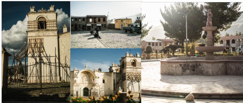
[Photo 9] Church and houses in collapse situation.
