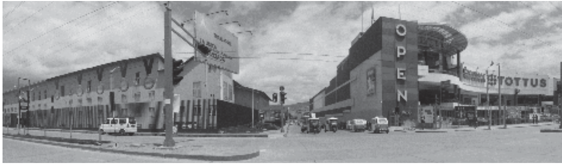
Figure 42: Open Plaza mall and the North Private University in the study area
