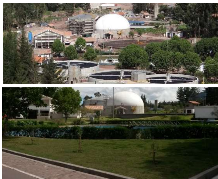
FIGURE 3.8 TOP: VIEW OF THE TFs AND SCs OF WWTP; BOTTOM: VIEW OF OSC (PHOTOS 2016)
